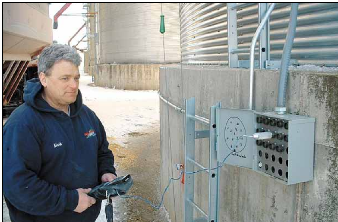
Checking grain temperatures is a weekly occurrence at Hull Coop. pictured: Mark Hoekstra, Grain Supervisor
